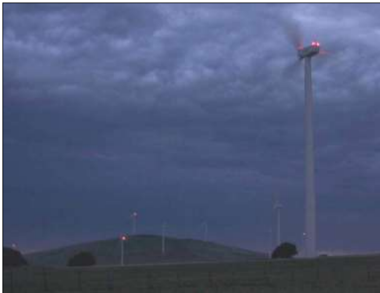
Photo 2: Warning lights and visual effects, blades emphasised by the lights
