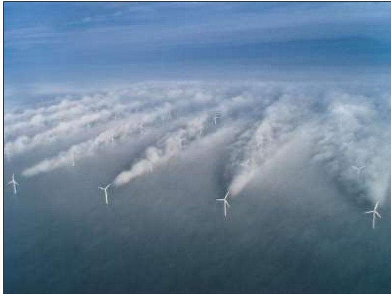
Figure 7: Horns Rev 1 Offshore Wind Farm 'Aeolus' turbulence behind the Horns Rev1 wind farm under very humid conditions, 12 February 2008 at 1300hrs. Photographer Christian Steiness
